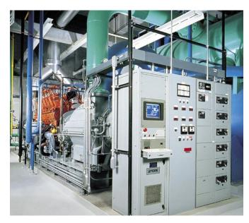
Critical parameters of the Titan chiller are monitored and controlled by industrial-grade, application-specific control systems to ensure reliable operation.
